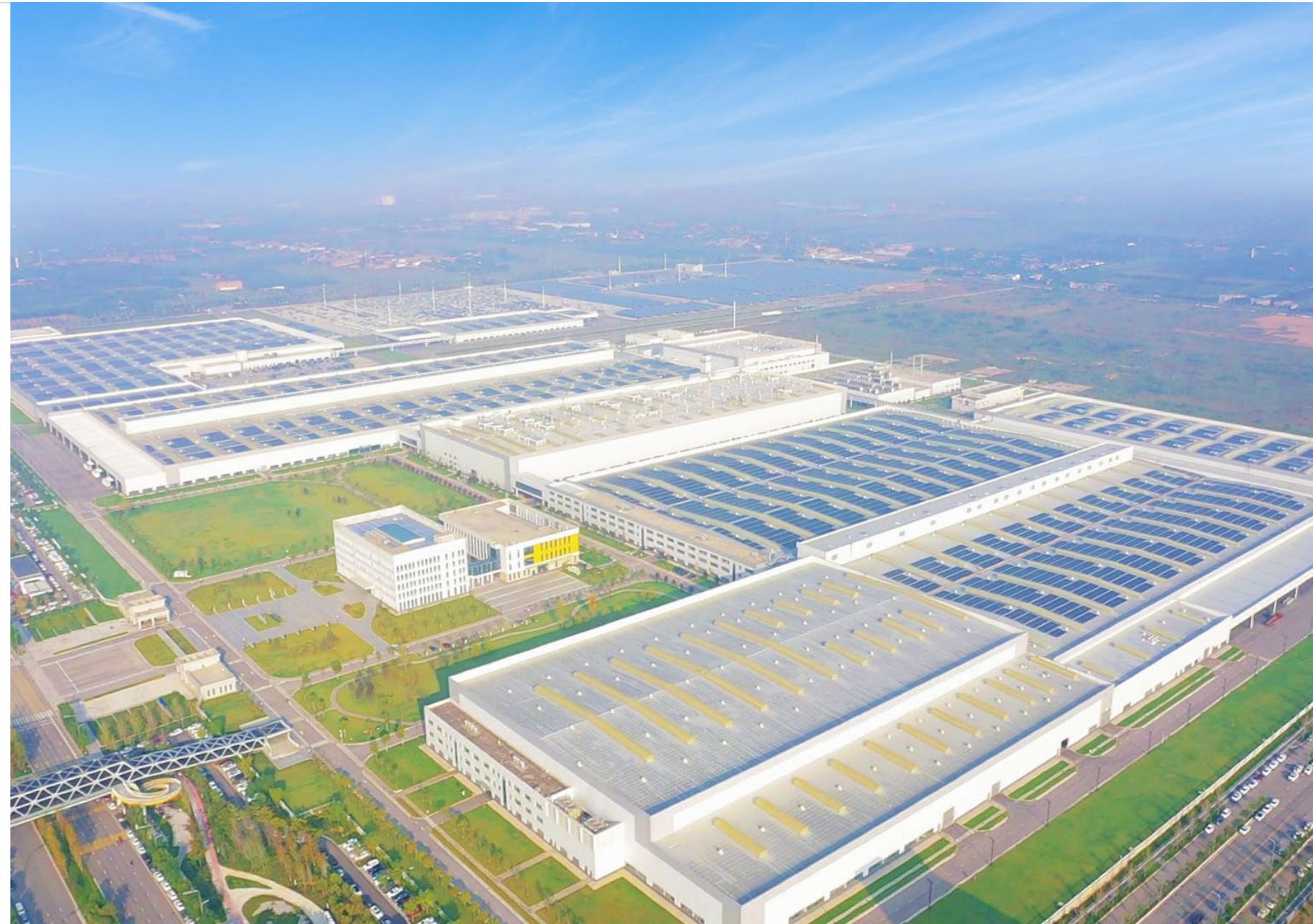
Photovoltaics power station at Geely Auto's plant
