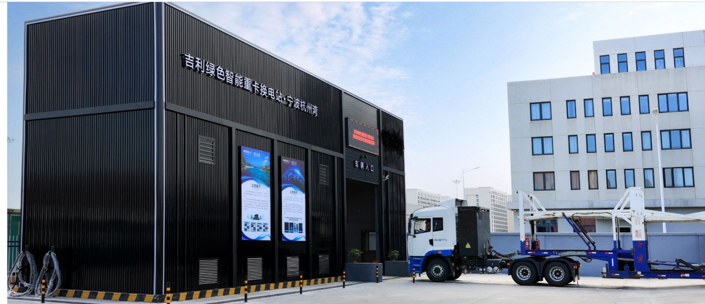
Intelligent green battery swapping station for heavy-duty trucks
